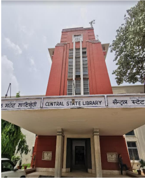
1. Image of the main tower of the library building. Image by author.
