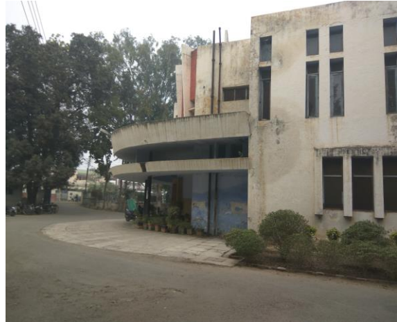
15. Side façade. Image from Google view.
