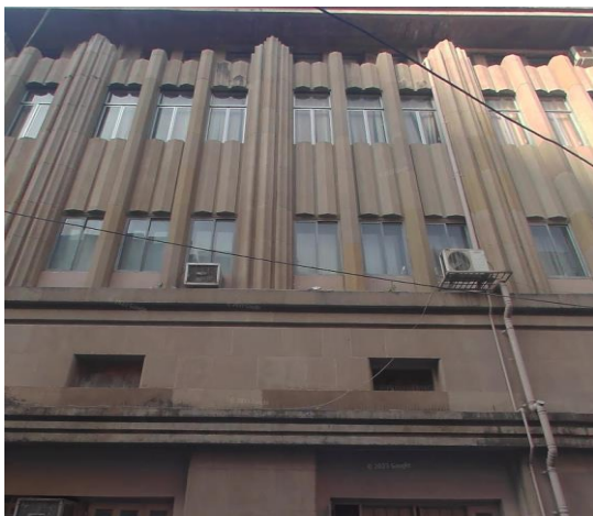
5. Image of the back elevation. Image from Google Street View.
