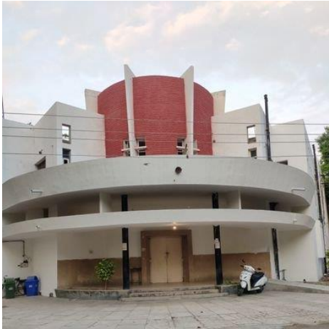
14. Front façade. Image from Google view
