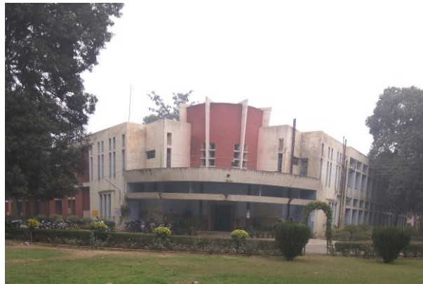
13. Whole building block. Image from Google view.
