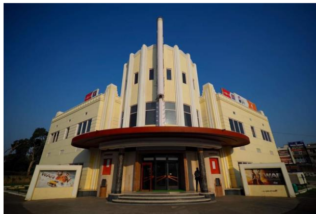
7. Front elevation of the building. Image by author
